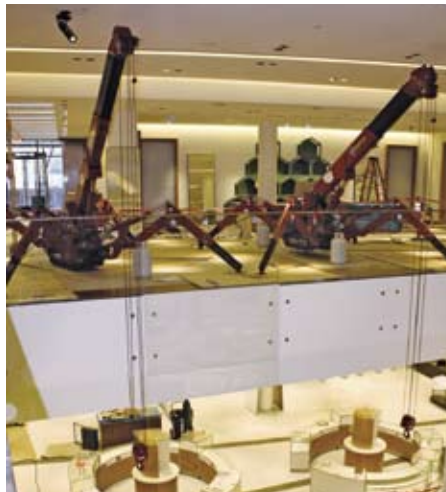
Non-marking tracks made SpyderCrane's Unic URW295 the crane of choice in installing a shopping mall staircase in Phoenix, Ariz.
